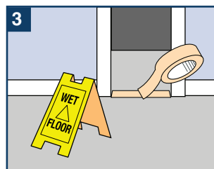
3 Tape off doorways and edges. Place wet floor signs at all entranceways. 10 - 15 Minutes
